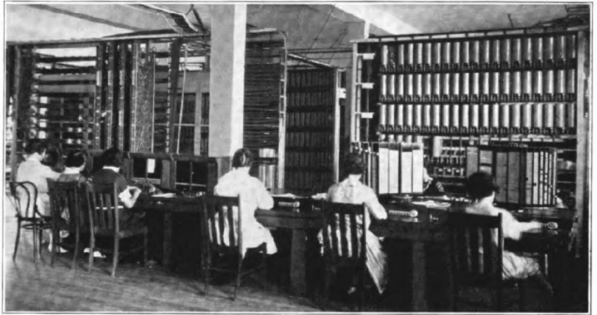
Main Office Switchroom Showing Information and Complaint Desks.
