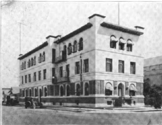
The New Main Office Building at Long Beach.
