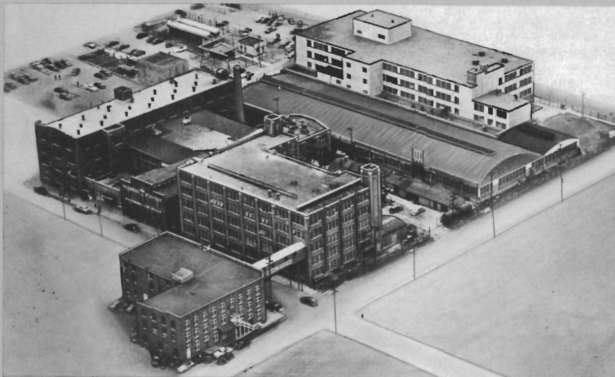
To meet requirements of the Armed Services for high-reliability tubes, General Electric enlarged its factories such as this one in Owensboro, Kentucky. By the middle of 1952, production of G-E Five-Star tubes was increased 5 to 1 over 1951.
